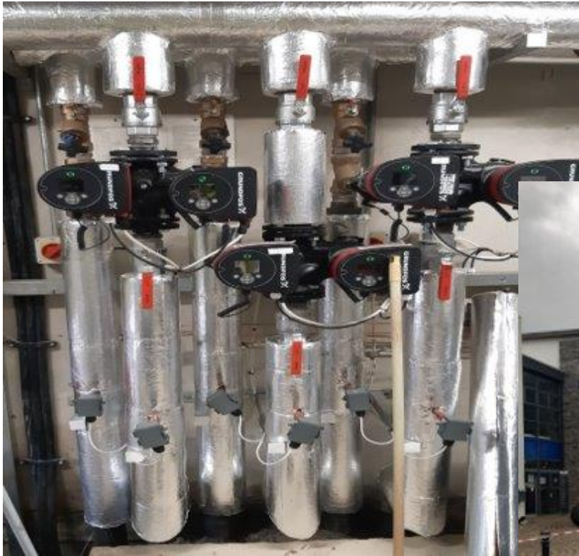
Pump Controls to BMS
