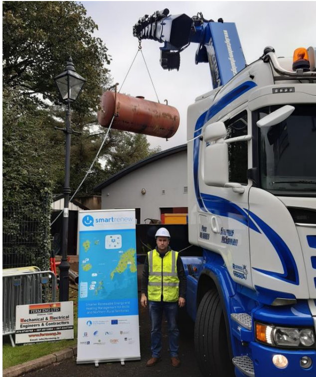
Oil Tank Removal
